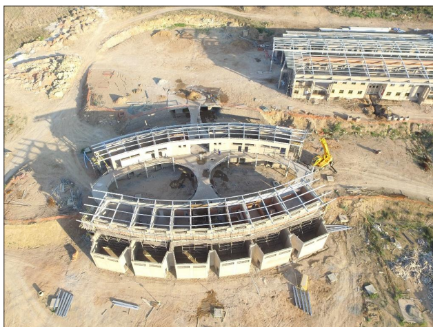
Fig. 4. The early stages of phase 1 construction of the WSU medical school.
