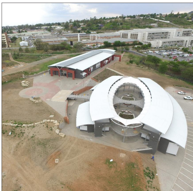
Fig. 5. Completion of phase 1 of the WSU medical school.
