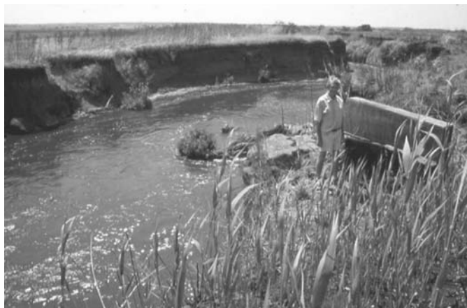
Fig. 5. Photograph showing the extent of channel incision at the inlet (concrete structure next to figure) to the irrigation pump shown in Fig. G. Figure G provides an aerial view of this location.
