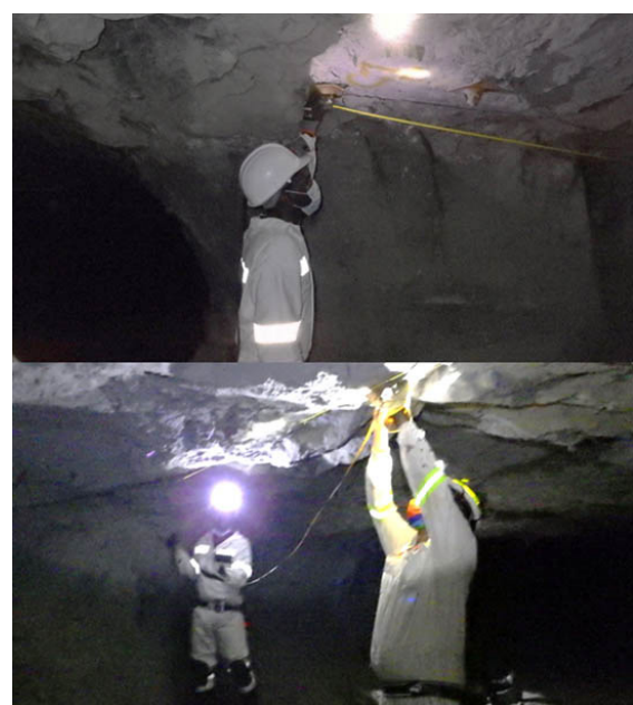
Figure 2—Roof bolts used as a reference point of the survey grid
