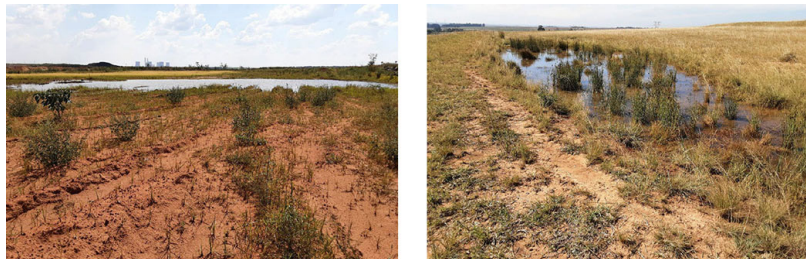
Figure 5—Water ponding observed during the site assessments
