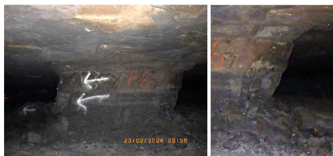
Figure 11—Pillar P92 photographed underground. Signs of spalling are noticeable in the right photograph
