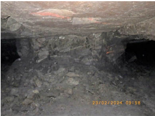
Figure 16—A pillar that is classified as failed, and it has a width-to-height ratio of 0.97
