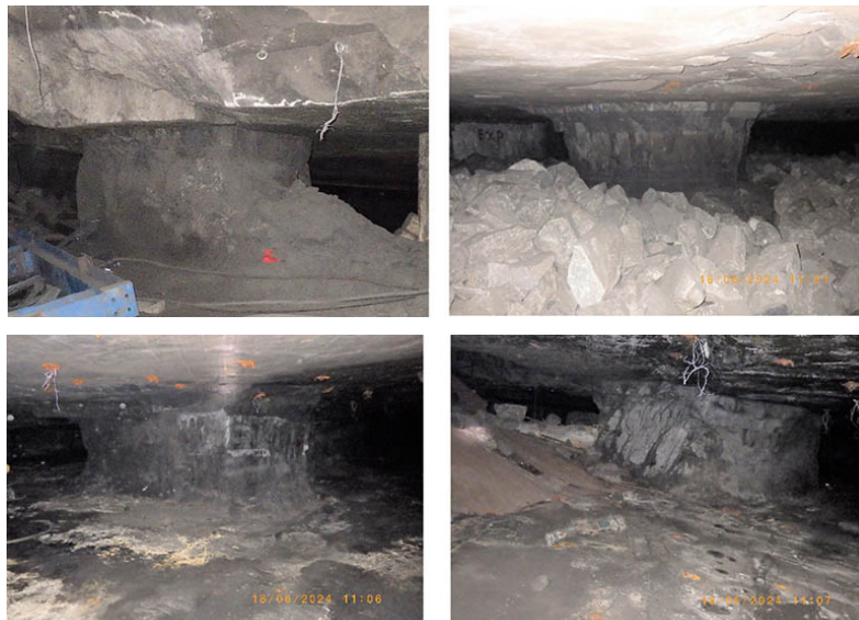
Figure 14—Photographs of some of the small pillars that were simulated using Map3D. Note that these pillars still appear stable in spite of their small sizes
