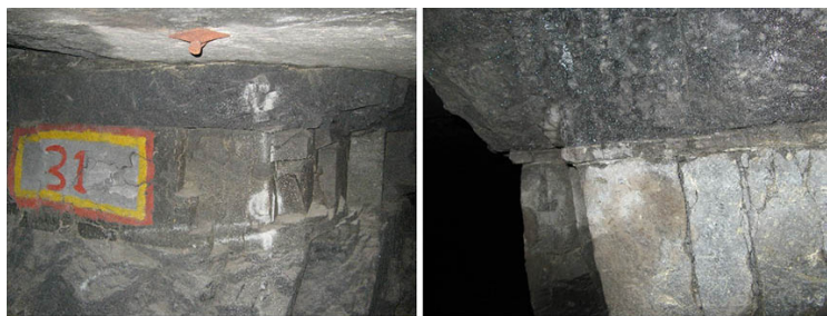
Figure 1 —LG6/LG6A pillars. Note the internal waste band comprising pyroxenite. A weak contact between the chrome and pyroxenite is shown on the right. The resulting pillar behaviour and strength are difficult to simulate using inelastic codes
