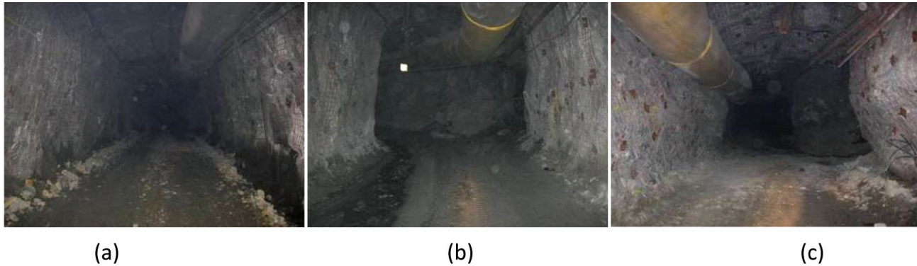
Figure 2 – Variations in squeezing severity in three locations less than 100 m apart at 2150 m depth, LaRonde mine. (a) Perpendicular – no squeezing; (b) 45 degrees – minor or no squeezing; (c) parallel – severe squeezing (after Mercier-Langevin and Hadjigeorgiou, 2011)
