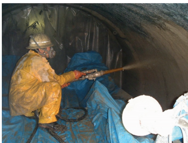
Figure 1—Typical mechanized sprayed concrete application
