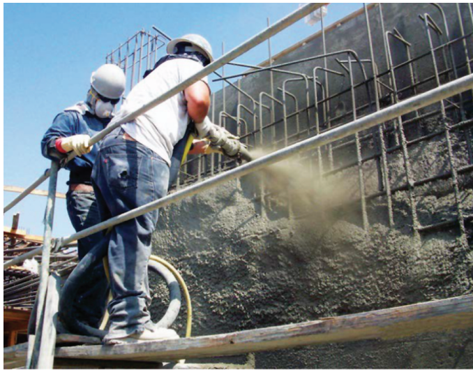
Figure 5—Typical hand-held sprayed concrete application
