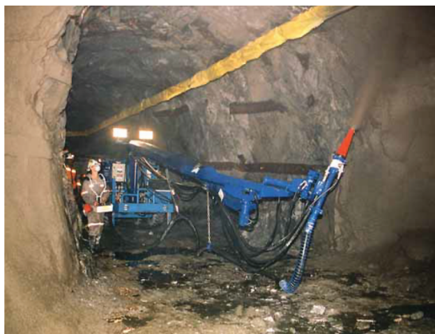
Figure 1—Typical mechanized sprayed concrete application
