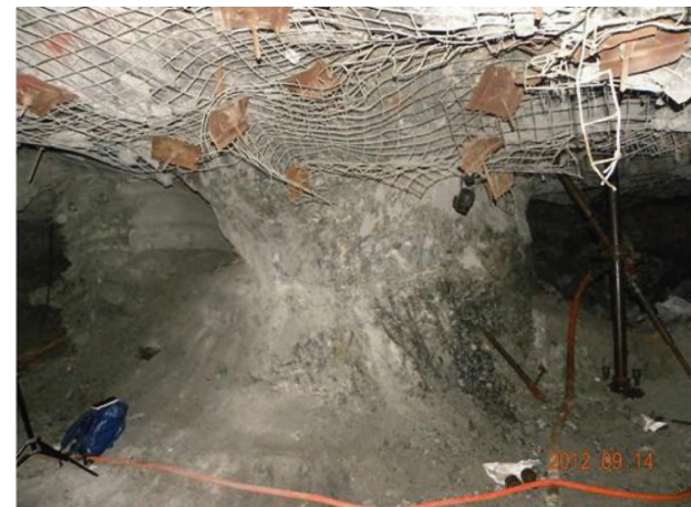
Figure 31—Pillar 1, which was instrumented soon after formation. No dynamic closure had occurred
