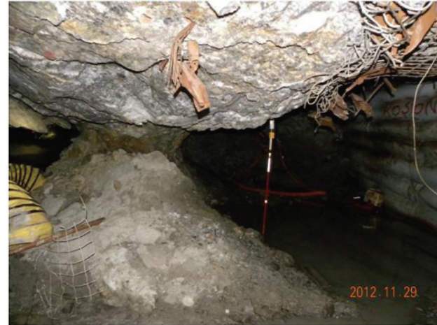
Figure 33—Pillar 2, stress measurements were conducted six months after formation. More than 300 mm closure, including some dynamic closure, had taken place
