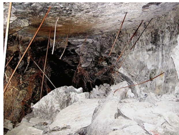
Figure 9—Co-seismic damage at a cubby along the southern sidewall of the tunnel 18 m below the on-reef pillar shown in Figure 8 (Case 3)
