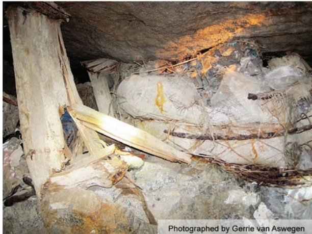
Figure 10—Crushed concrete pack next to the pillar that failed (Case 3). Total dynamic closure exceeded 110 mm
