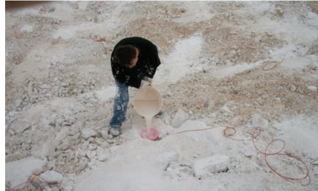
Figure 1—Application of plaster paste to hole collar
