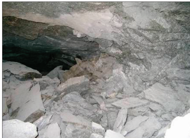
Figure 12—Up-dip side of Pillar 16
