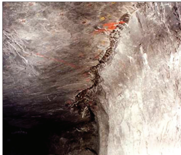
Figure 2—Roof guttering at the pillar-roof contact
