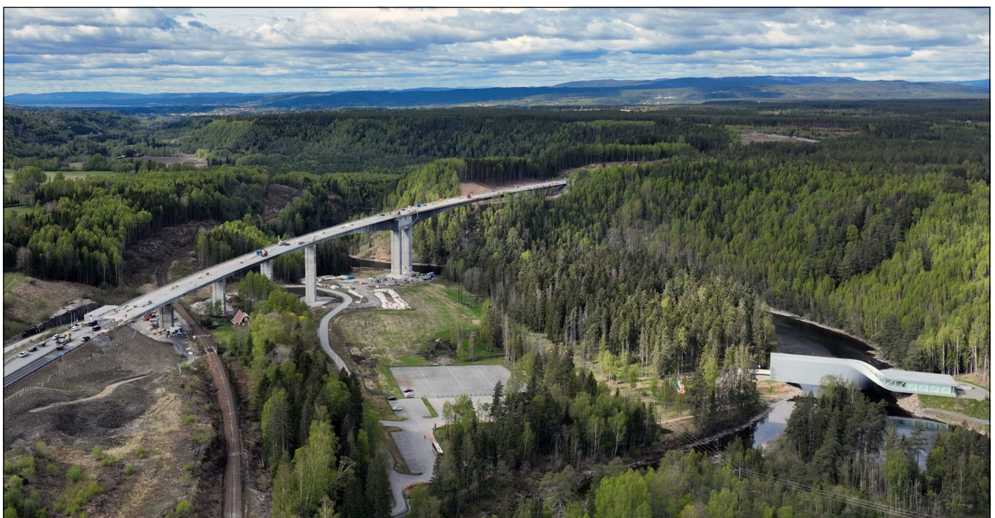
Figure 6 Randselva Bridge, currently the world's longest bridge built without drawings using BIM (Savland et al 2022)
