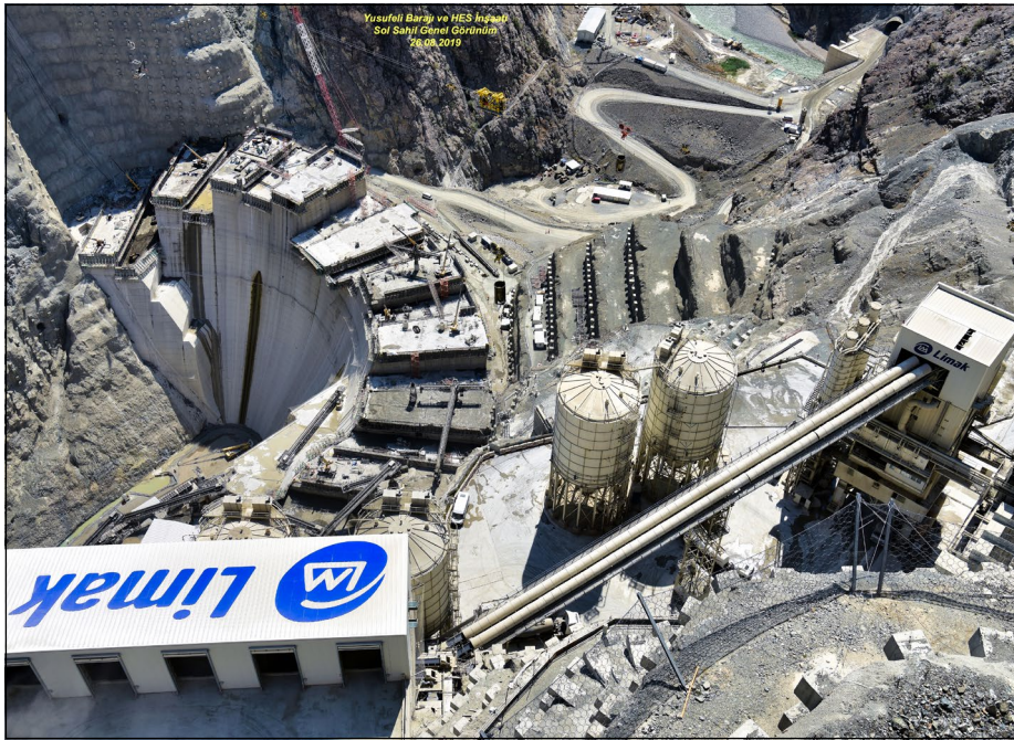
Figure 5 View of concrete construction works showing batch plant and cooling plant on left abutment (26 August 2019)
