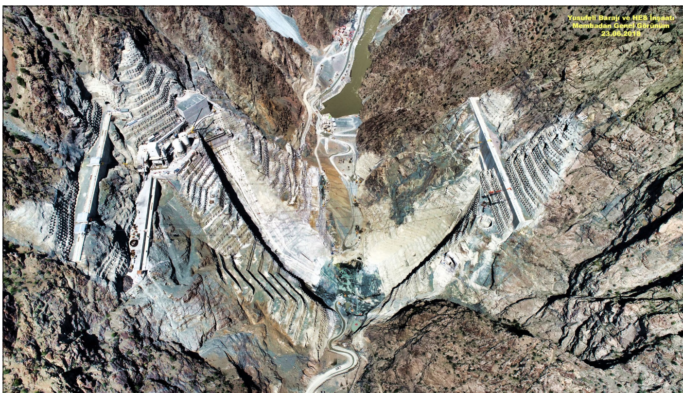
Figure 4 View of foundation excavation looking down stream (23 June 2018)
