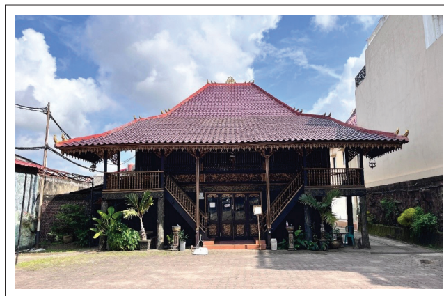
Source: Arni, Y., Fitri, E. A., Rahayu, C., & Darsin, D. (2025). Stilt house roof, [Photograph]
