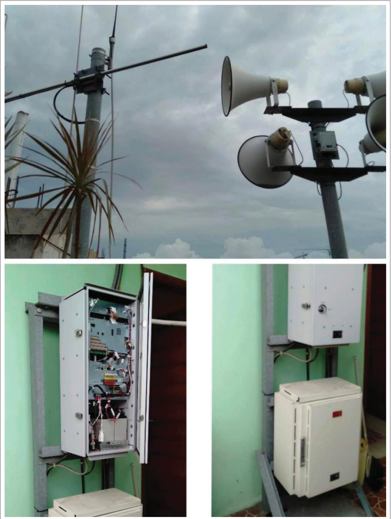
FIGURE 6: Disaster early warning system (DEWS) for a flood at Rawa Buaya Urban Village.
