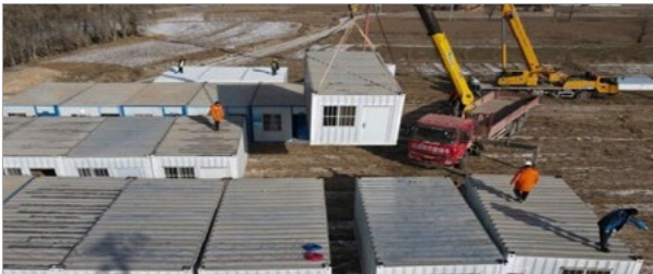
Figure 3: Temporary housing units in Meipo Village, Jishishan County
