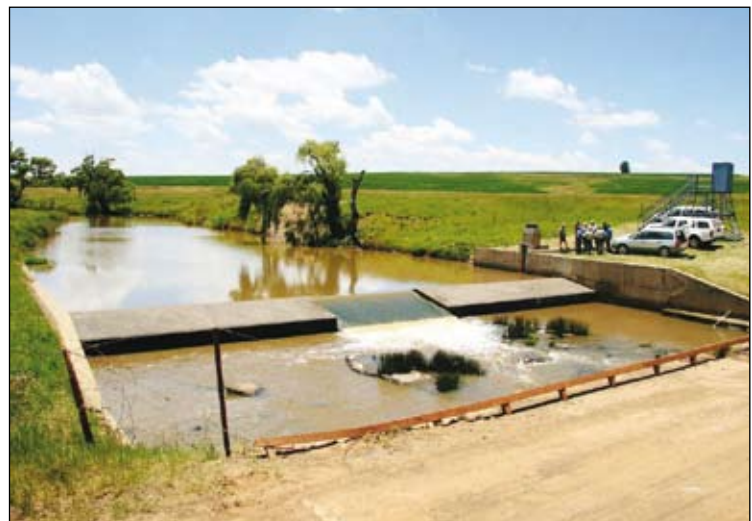
Figure 9 Example of a horizontal compound Crump weir without dividing walls in the Vaal River catchment (Mpumalanga)
