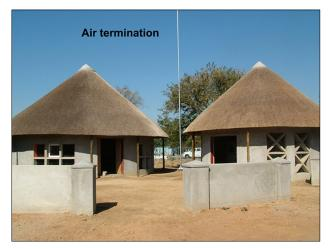
Figure 3: Thatch roof housing structures with single-mast lightning protection system.
