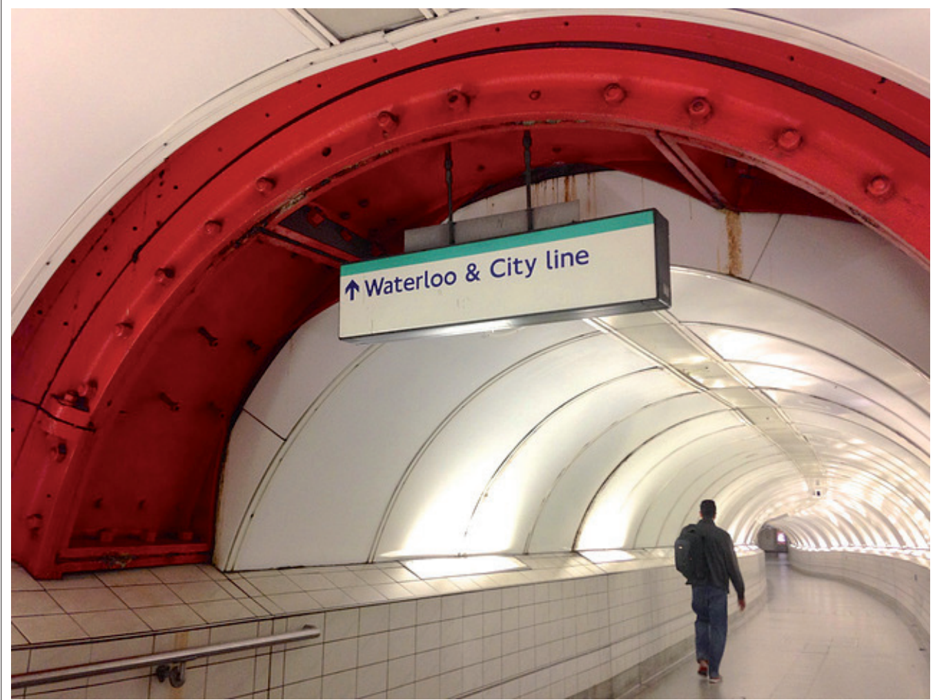
FIGURE 14: Bank Station: Remains of a discarded Greathead Shield used in building the Waterloo and City Line.
