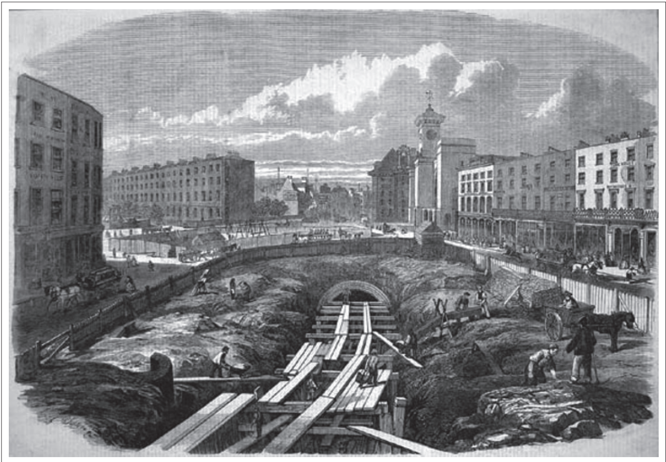
FIGURE 10: Cut-and-cover construction on the Metropolitan Line, the world's first underground railway, which opened 10 January 1863. Wooden, gas-lit carriages, hauled by steam, carried passengers between Bishop's Road, Paddington, and Farringdon.
