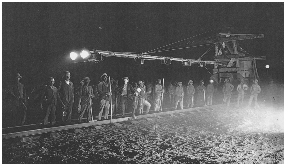
Figure 12: '[A]n innovative contraption generating electric power for floodlights to facilitate night working – Prieska' (Transnet Heritage Library, Johannesburg).
