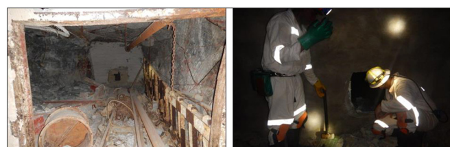
Figure 13—Opening sealed off workplaces
