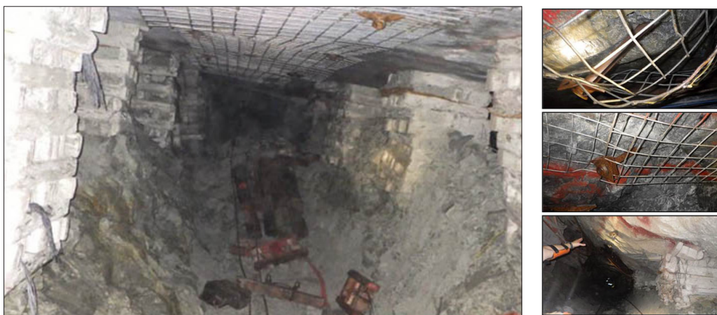
Figure 14—General gully excavation and support conditions
