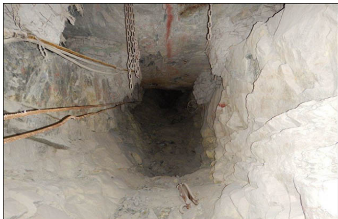
Figure 6—Historical practice - no rockbolts or mesh installed along the gully hangingwall
