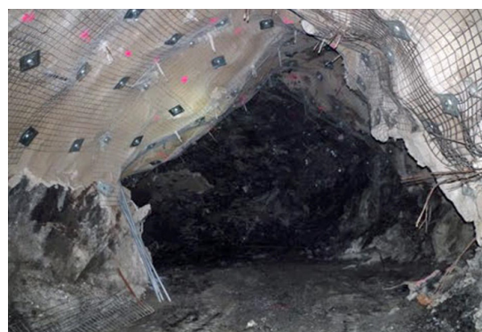
Figure 14—Agnew gold mine drive after rehabilitation, (Andrews, 2019)
