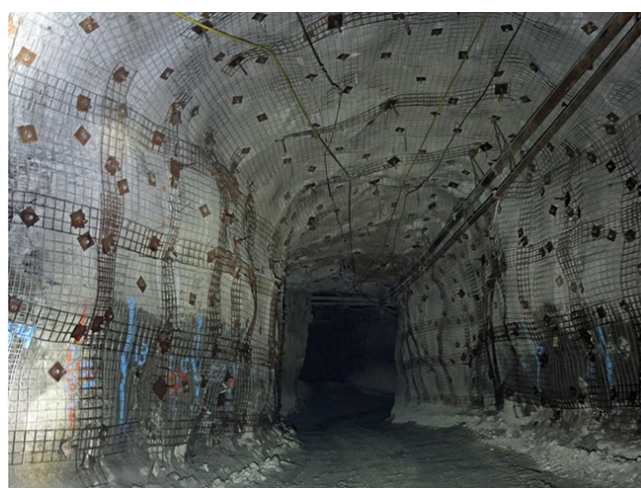
Figure 7—Installation of ground support close to the floor
