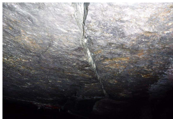
Figure 8—Tensile cracks in the hangingwall of the level 5 failure zone
