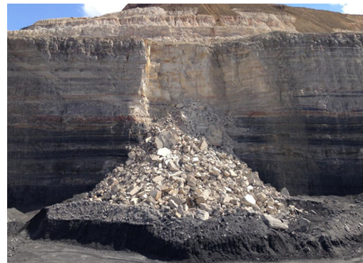
Figure 1—Slope failure with wedge-style back scarp failure mechanism
