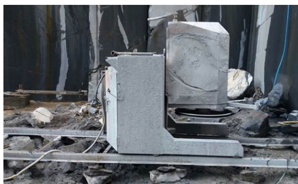
Figure 2 —Diamond wire saw machine on surface track
