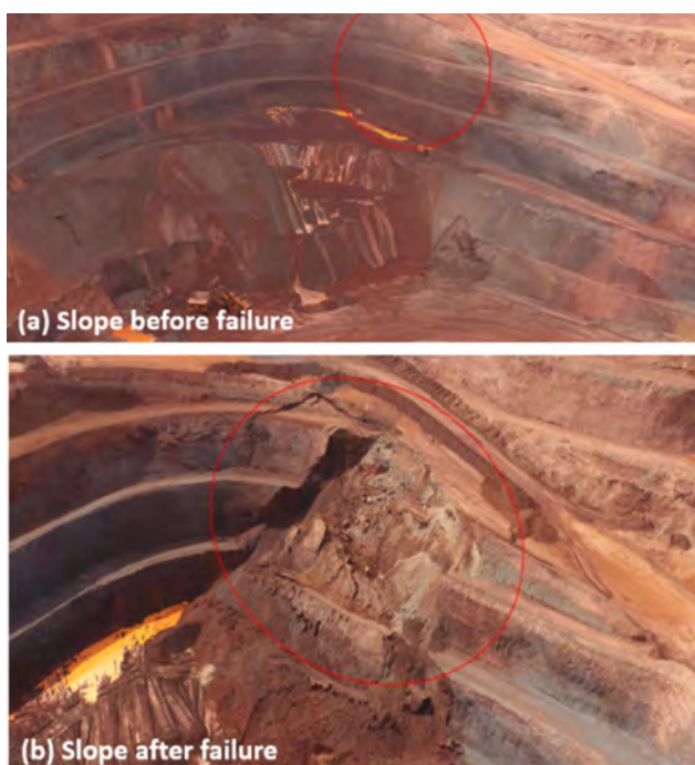
Figure 2—Slope failure 2018
