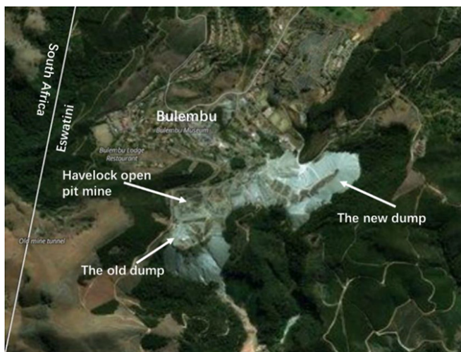
Figure 2—Aerial view of Bulembu and location of the TSFs
