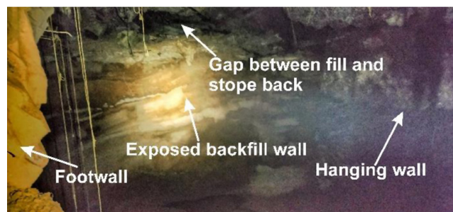
Figure 10—Exposed cemented hydraulic fill wall in the chromite mine
