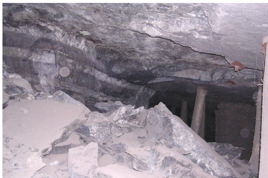
Figure 8—Down-dip side of Pillar 8. View away from panel face
