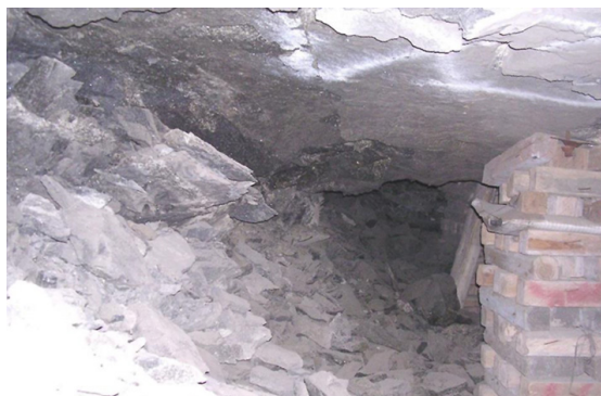
Figure 10—Down-dip side of pillar 3
