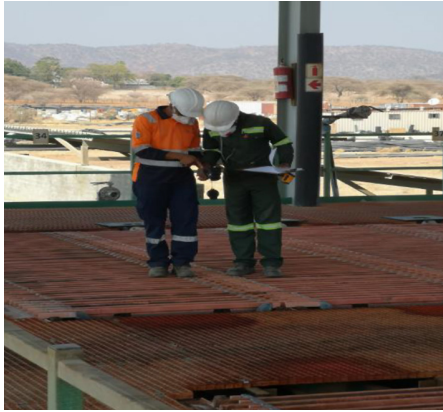
Figure 5—Detecting hotspots using an infrared (IR) camera
