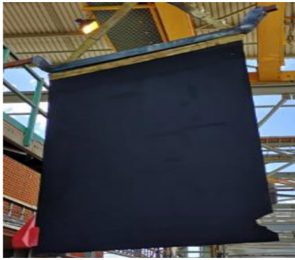
Figure 11—Replacing an anode with a missing side insulator
