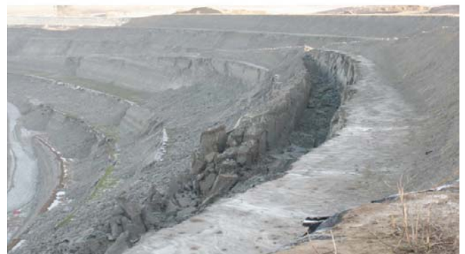
Figure 27—Toppling in 2010 following heavy rains. The installation of topsoil and plastic sealing can be seen in the lower benches in the distance
