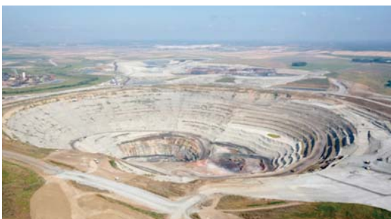
Figure 20—Configuration of the pit in late 2012. Note the weathered condition of the older phase 1 area in comparison to the more recently constructed slopes on the right
