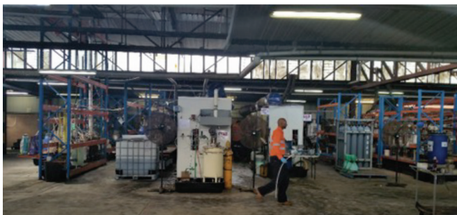
Figure 6—Integrated Kell pilot plant in 2016, showing 100 L long-term materials of construction testing system in centre foreground (photo with permission of Simulus)
