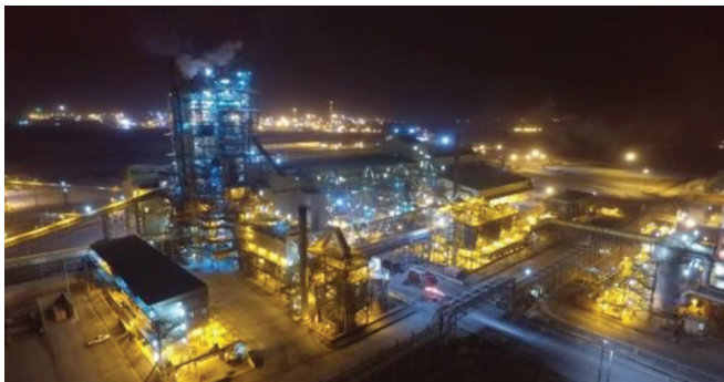
Figure 1—Night photograph of the KMP smelter. The tallest structure at the top left houses the Isasmelt furnace, with the MSEF located to the right on the ground level. The existing KMP mining and processing sites are seen in the background
