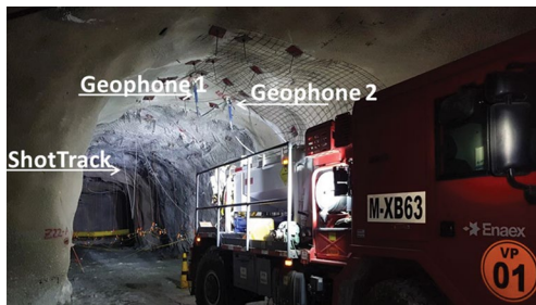
Figure 9—ShotTrack cable and charged holes (Paredes and Rodriguez, 2018)
