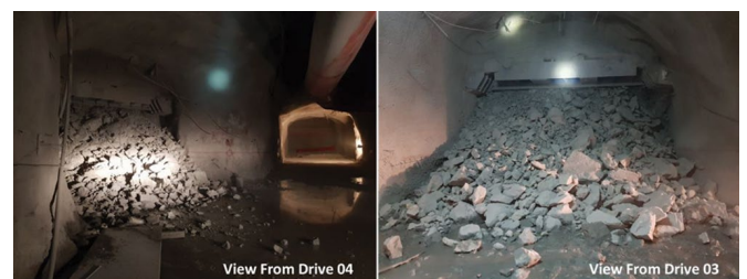
Figure 24 – Blasted material pile in drifts 3 and 4. drawbell 2 (Paredes and Rodriguez, 2018)
