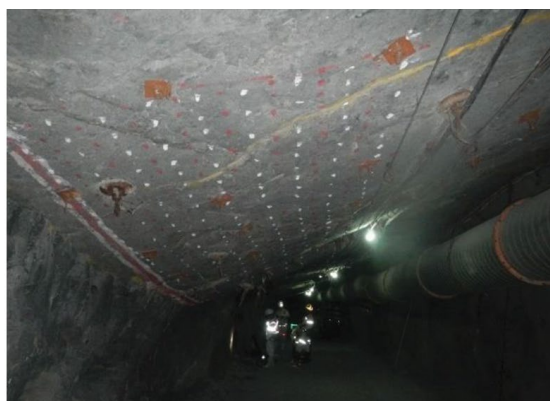
Figure 5—Hangingwall survey block at Mine B. The grid of white spray paint markings was used to guide data acquisition
