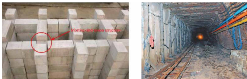
(a) Mortise and tendon hollow wall made of concrete block (Luan et al. , 2018)
