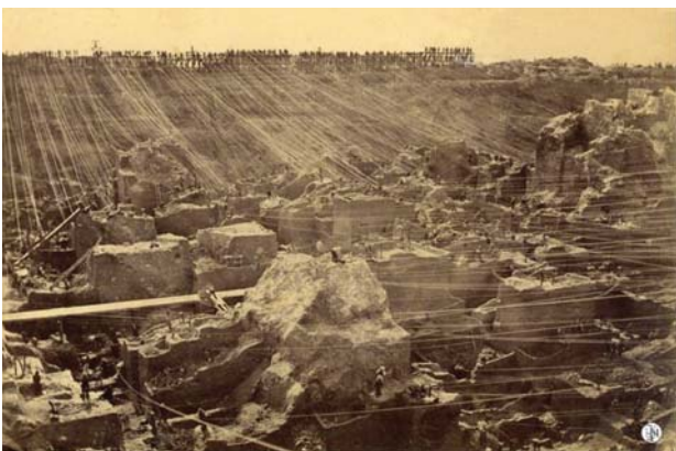
Figure 1—Little cooperation between diggers is illustrated by the numerous ropes from 'stages' to claims ( http://www.milnerlodge.co.za )
