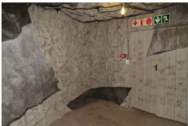
Figure 8—This figure shows the fault intersected in the tunnel spur. The dark coloured lithology on the left is the UG2, while the dark coloured lithology in the centre is the UG1. If the model is not manually corrected, the UG1 does not intersect the spur (as found in the tunnel) but is rendered deeper in the footwall (2017)
