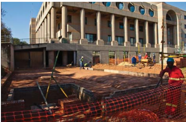
Figure 1—Construction of the Wits Mining Tunnel in 2013
