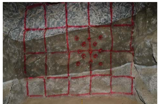
Figure 9—This figure shows the face of the main portion of the tunnel. The dark lithology observed is the UG2. If the model is not manually corrected, the UG2 is rendered above the face of the tunnel (2017)
