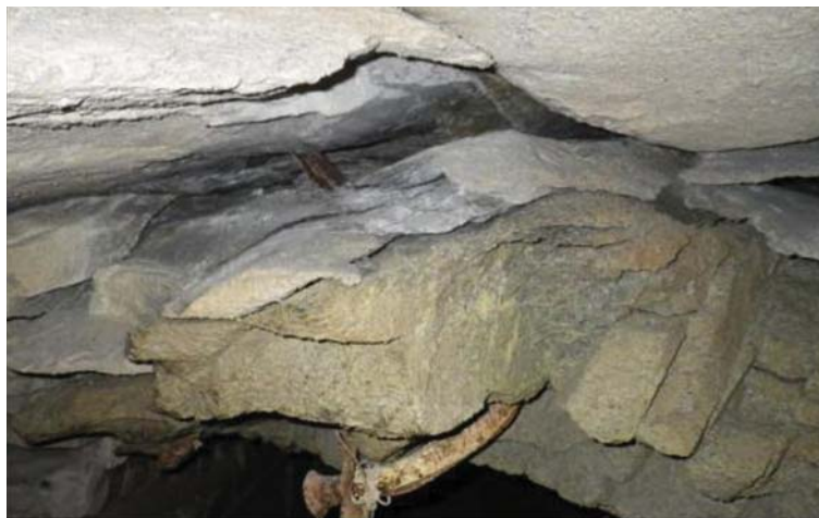
Figure 21—Unravelling of the hangingwall in the back area of the Libanon stope where the effects of the multi-reef mining could be observed. This damage can possibly be attributed to the tensile zone in the hangingwall caused by the de-stressing process
