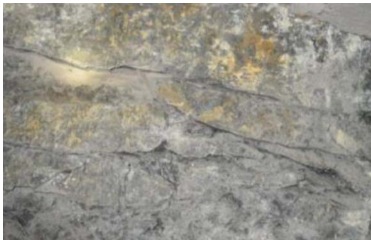
Figure 20—Condition of quartzite between the two reef elevations as seen in the sidewall of a newly developed orepass underneath the stope (in supposedly de-stressed conditions)
