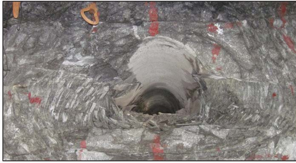
Figure 12—Photograph of exposed reef raise face, revealing extensive fracturing beyond the extent of breakout around the hole
