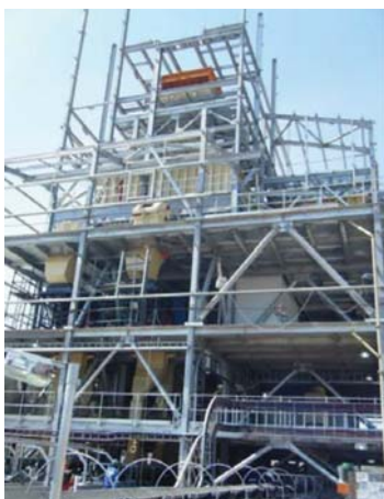
Figure 8—Karowe's XRT section during construction in Q2 2015
