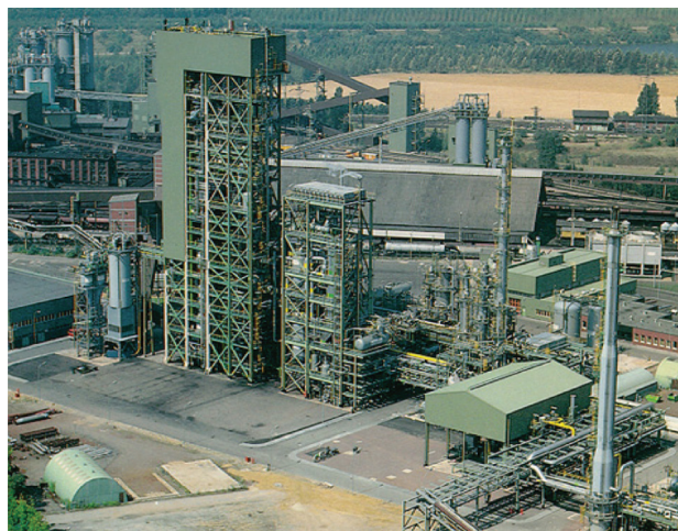
Figure 5 – HTW demonstration plant, Berrenrath, Germany. Production rates: 300 t / d methanol, total operating hours: 67 000 h (Renzenbrink et al., n.d)
