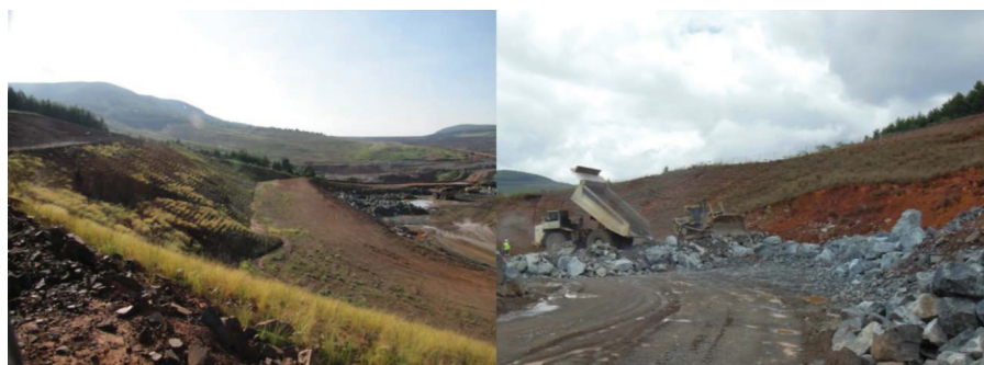
Figure 6—Comparison of the slope toe in 2010 (left) and in December 2012 (right)
