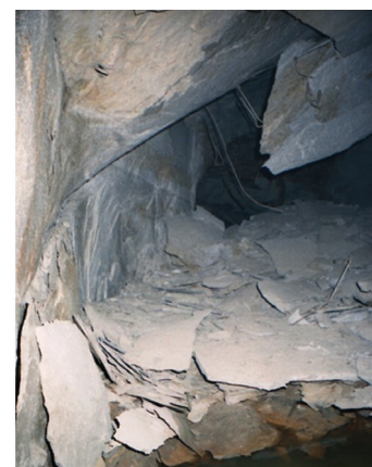
Figure 4—Stress-induced failure in the roof of a dip-oriented tunnel in a platinum mine (Stacey and Wesseloo, 2004)
