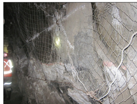
Figure 3—Spalling in a haulage tunnel in a platinum mine, western limb, Bushveld Complex
