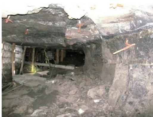
Figure 9—Delamination of hangingwall in a platinum mine stope
