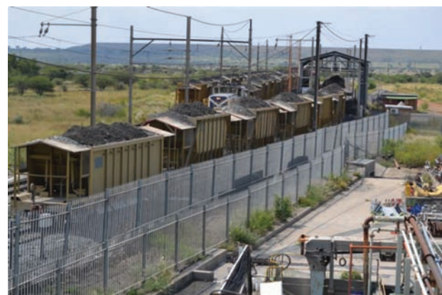
Figure 2—Span of hoppers en route from shaft to plant
