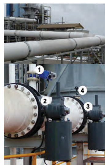
Figure 6—Pipeline for sulphuric acid-containing off-gas. Motor-driven butterfly valves (1-3) and temperature sensor (4) courtesy Plastilon OY, Finland)
