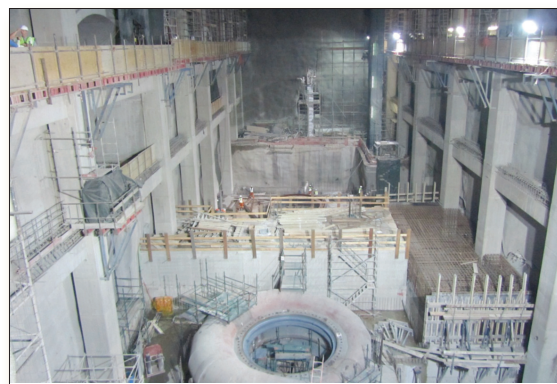
The Machine Hall of the Ingula Pumped Storage Scheme under construction
