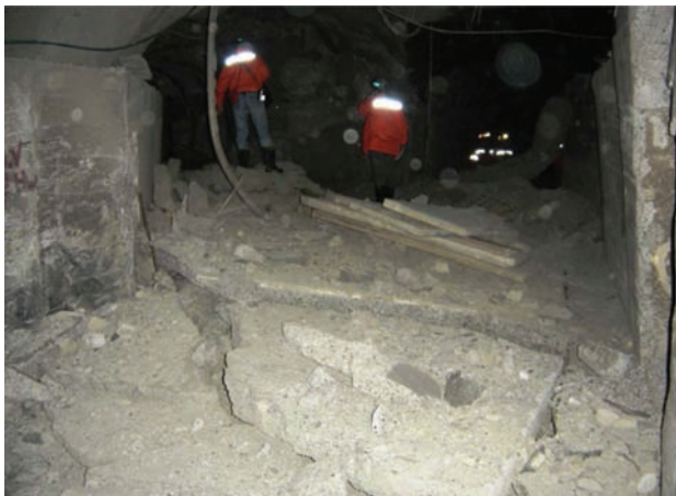
Figure 2—Floor heave of nearly 2 m caused by a rockburst (photograph T.R. Stacey)
