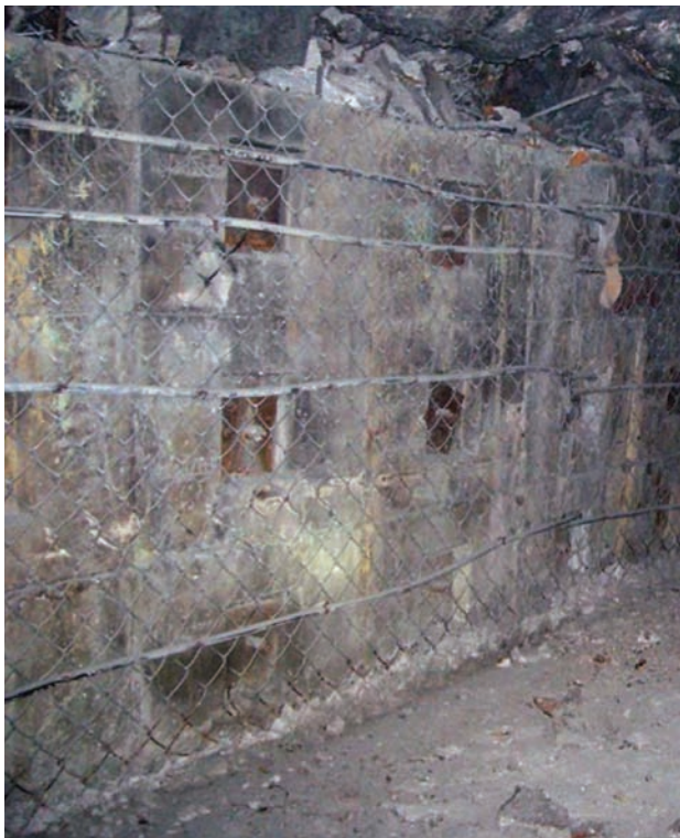
Figure 16—Remedial 'staple' support with wire ropes (photograph Y. Potvin)
