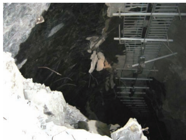
Figure 4—Upwards ejection of sidewall rock to impact service tray (photograph T.R. Stacey)
